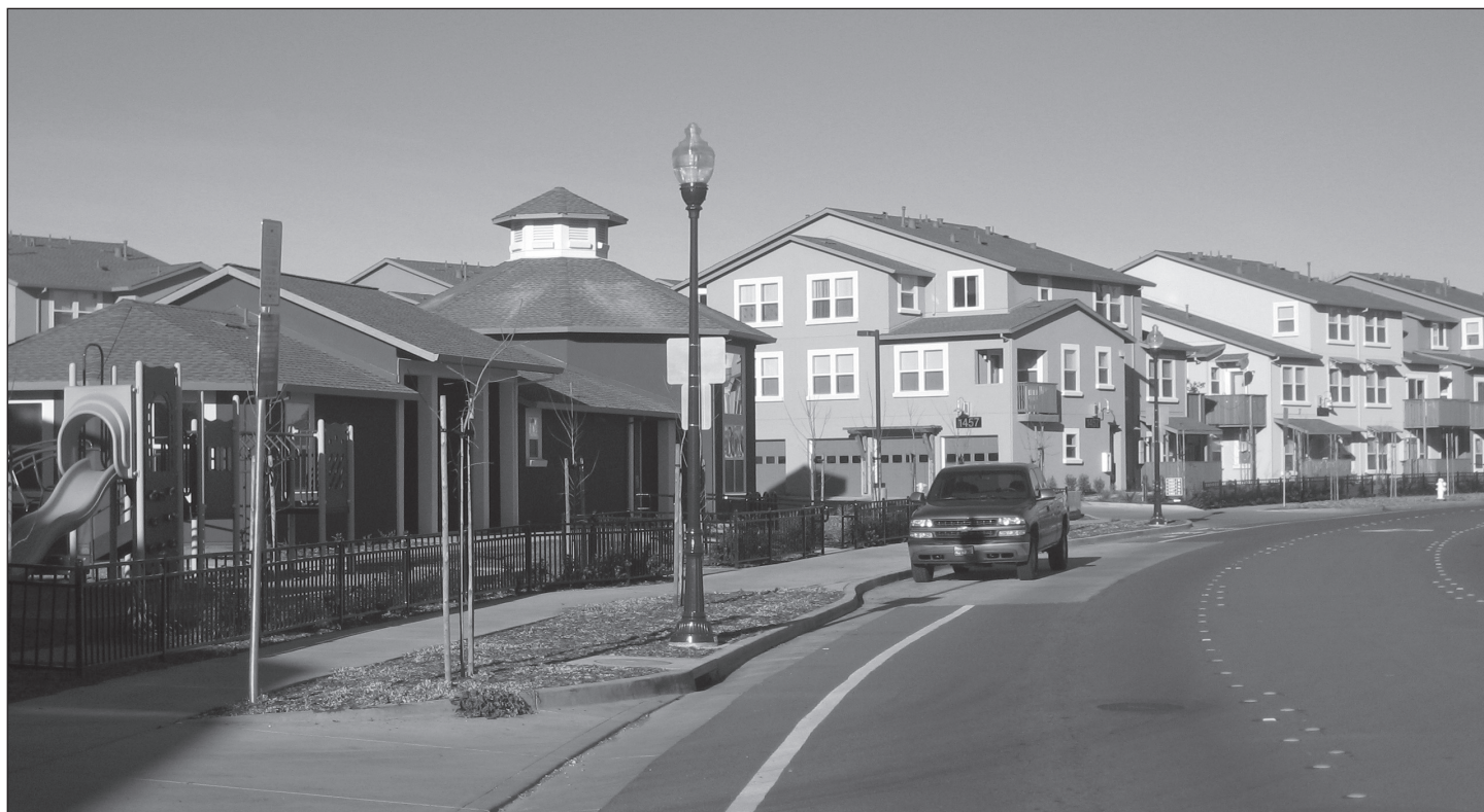
Burbank Housing used tax credits for this low to moderate density suburban development in Santa Rosa, California. The development included community facilities (photo by Tony Gilmour).
