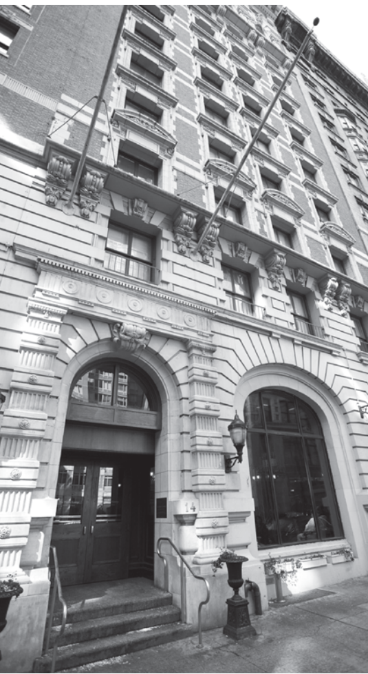
The Prince George, Manhattan, provides 416 units for formerly homeless people and those on low incomes. Part of the running costs is met by renting out the meticulously restored Prince George Ballroom. (Photo courtesy of Common Ground NY).
